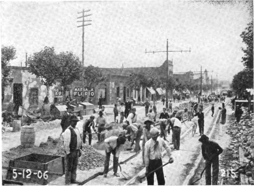
LAYING TEMPORARY TRACK FOR TRAMWAY LINE IN THE CITY OF BUENOS AYRES
